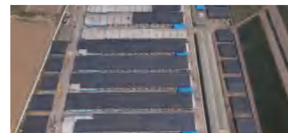
Qingdao Jiulian Project
